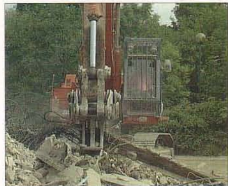
Demolition costs came to around £750,000
