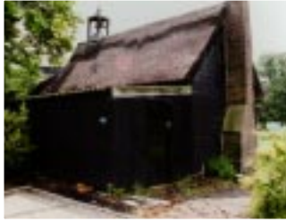
THE CHAPEL BEFORE RESTORATION
