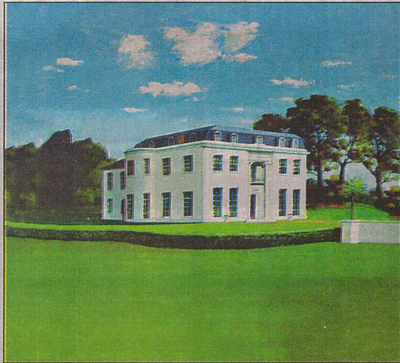
● PART OF HISTORY: Baldwyns Mansion is being restored
