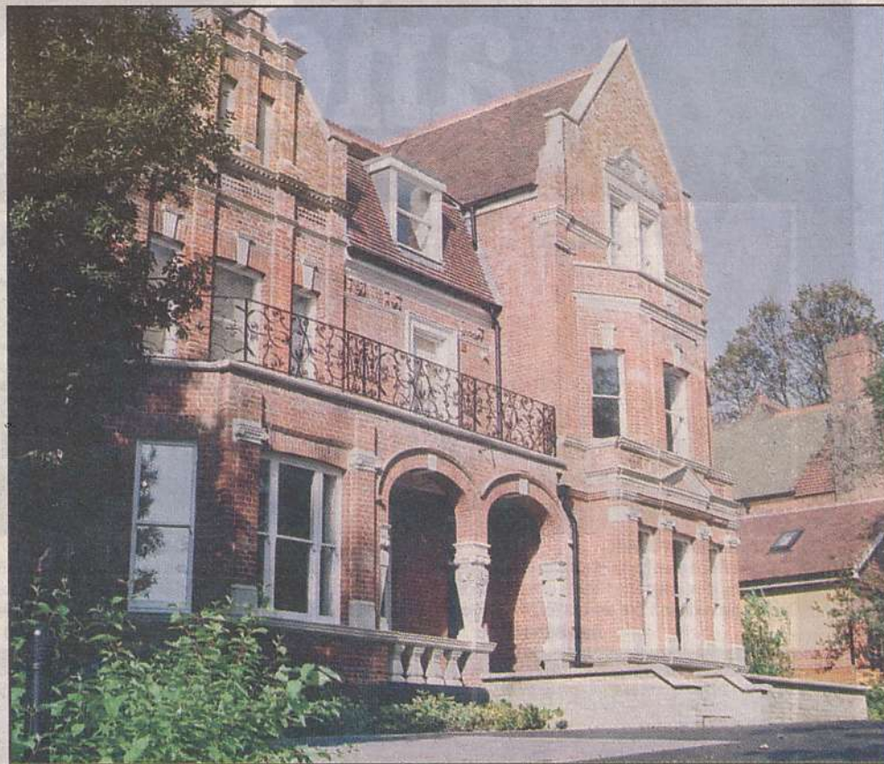
● The front façade of 15 Sundridge, a scheme by Morgan Restoration in Bromley
